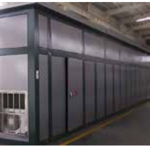
Compact Prefabricated Substation
