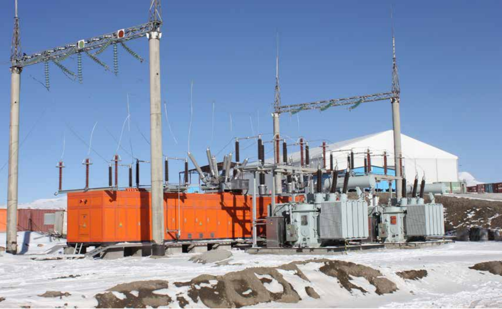
Compact Prefabricated Substation
