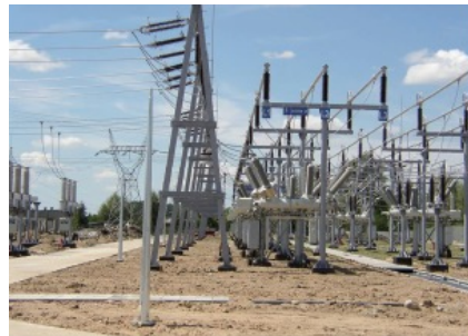
Double busbar arrangement
